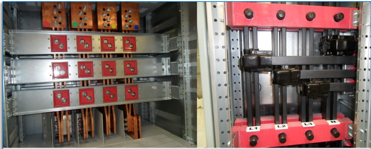
Figure 5.11 Non-Shrouded and Shrouded Bus Bars
